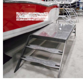
These boarding steps are an unprotected risk to boat show visitors: no railing!
