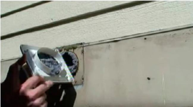
Before replacing the cover, return to the dryer, plug it back in, and run it on fluff. This will help blow out any loosened lint. After about 10 minutes, turn the dryer off, place the cover back on the outside vent and re-caulk the edges to keep out drafts.
