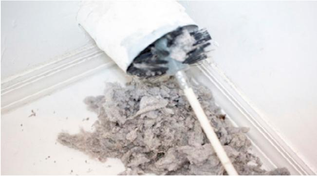
Clean as far down as possible. To clean even deeper, use a brush with a long, flexible handle (up to 10 feet long). Work the brush up inside as far as you can go. The brush will latch onto the lint and drag it out of the vent pipes.
