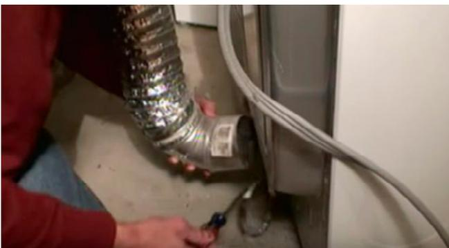
Dryer vents can get clogged with lint, which could keep your dryer from functioning properly.
